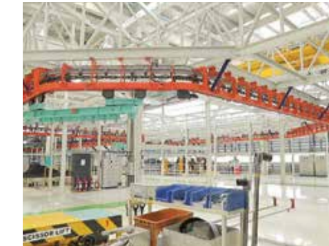
White paint on pillars and floors and use of natural light to reduce power consumption
