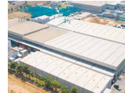
Double folded metal roofing for thermal insulating effects
